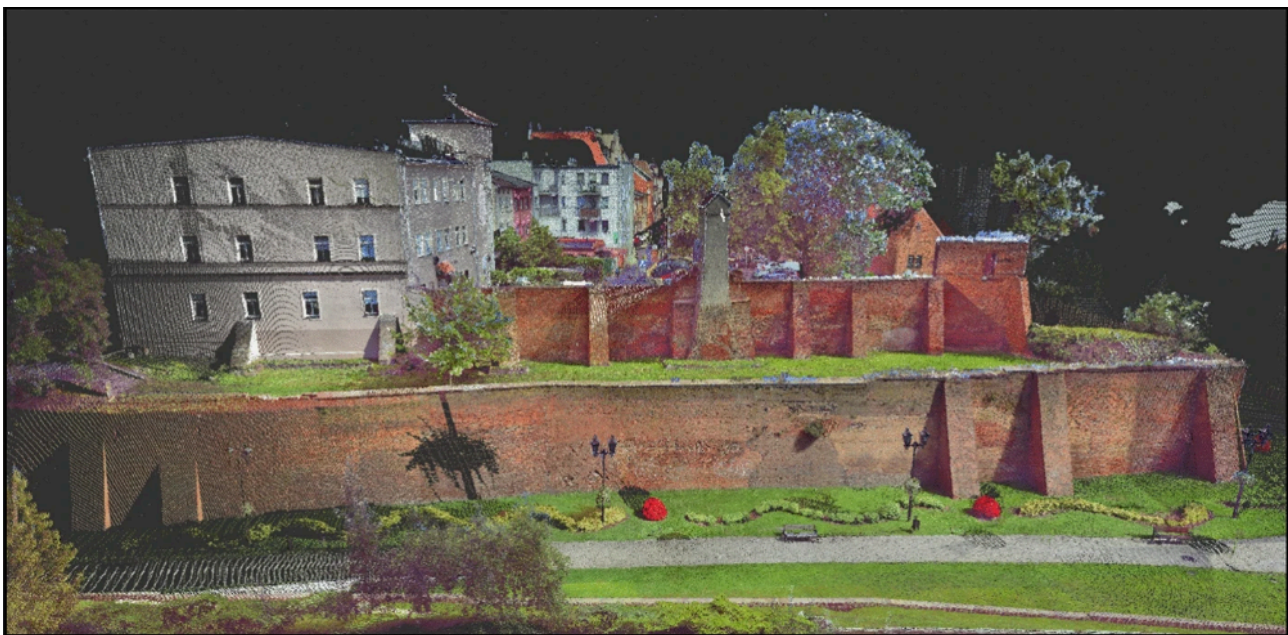
Figure 3: Digital model of a fragment of the southern section of the town wall in Grudziądz with the water tower (point cloud)
